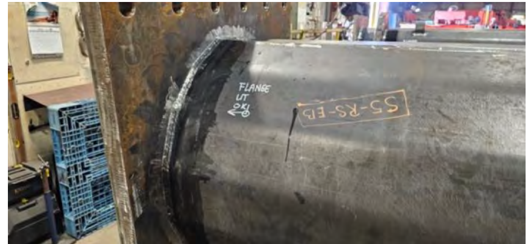
Welding and Inspection Complete (Longitudinal Seam & Baseplate Welds)
