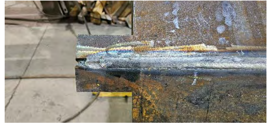
Visual Weld Inspection
