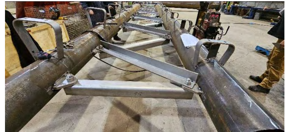
Fit Up Verification
